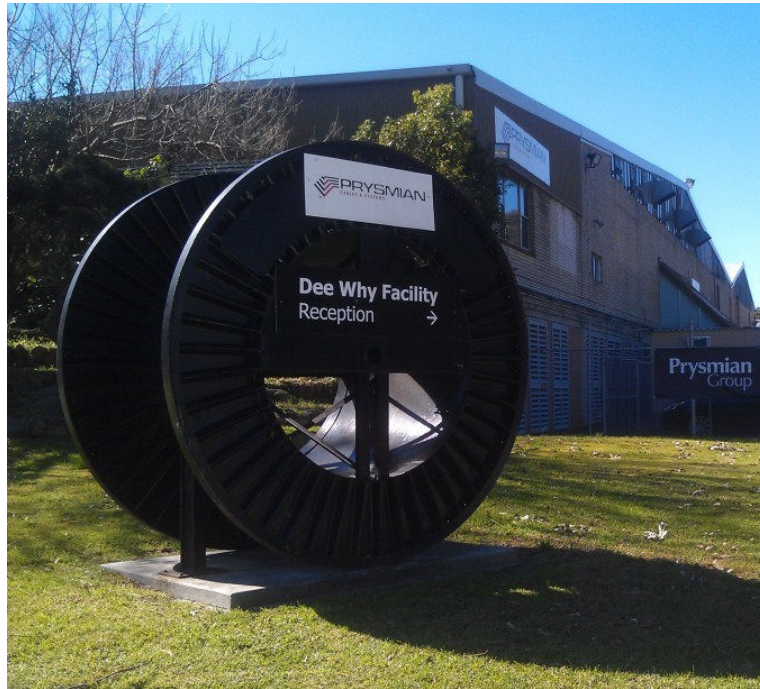
Dee Why, NSW Cable Manufacturing Facility
